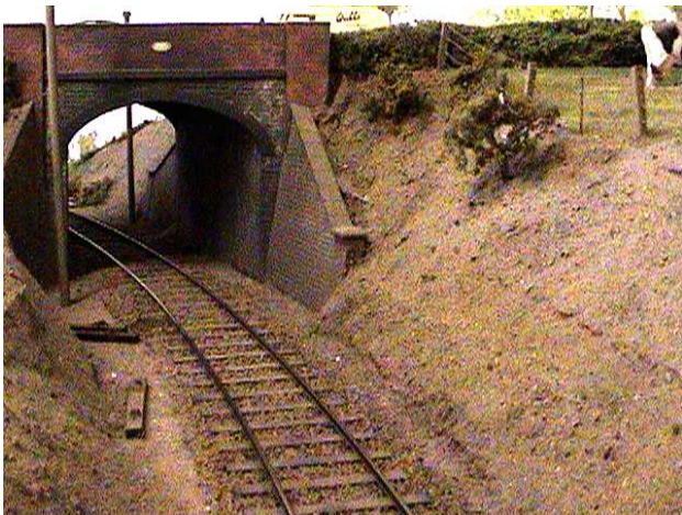
The road bridge
